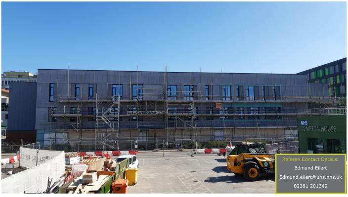
The works comprised of the construction of a two storey structure (Levels B & C) on top of an existing single storey building (Level A) which has been constructed to receive vertical expansion.
